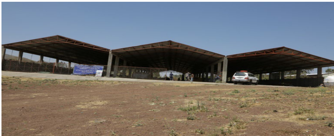
Compost Shed Bishoftu
