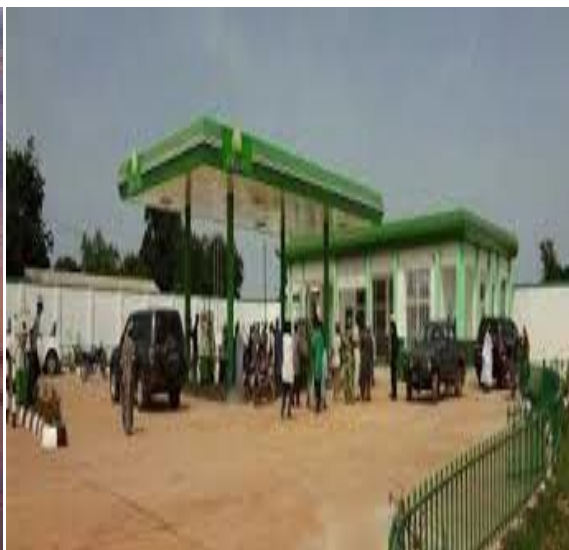
Gambia National Petroleum Company (GNPC) (Adjacent Fuel station)
