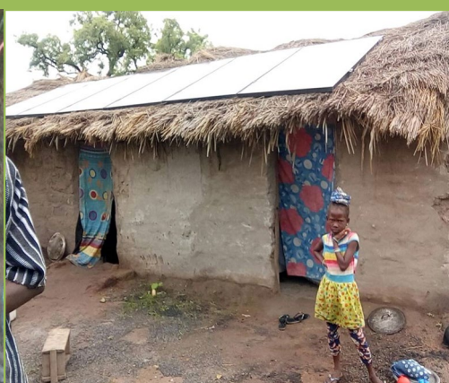
Solar Panels mounted on Hasimu's roof top
