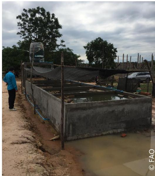
Picture 1: Fish hatching pond just completed cement plastering in Xonnobuly District. Need to leave tank filling water for some time before using it. The nursery pond recently dug very muddy water from the rain. Need to work on the pond to maintain clean water before releasing fish.
