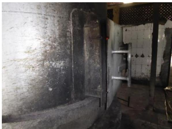
Waste is fed into the combustion chamber through this door
