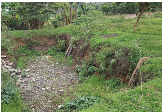
c. Coffee-washing infiltration ditch installed by the Burundi sustainable coffee project in Mwkiro community, 2015-17
