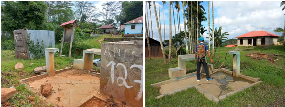
Photo 7: One water collection point that has stopped working (left) and another one that is fully operating near the water source (right) in Talimoro (Ermera)
